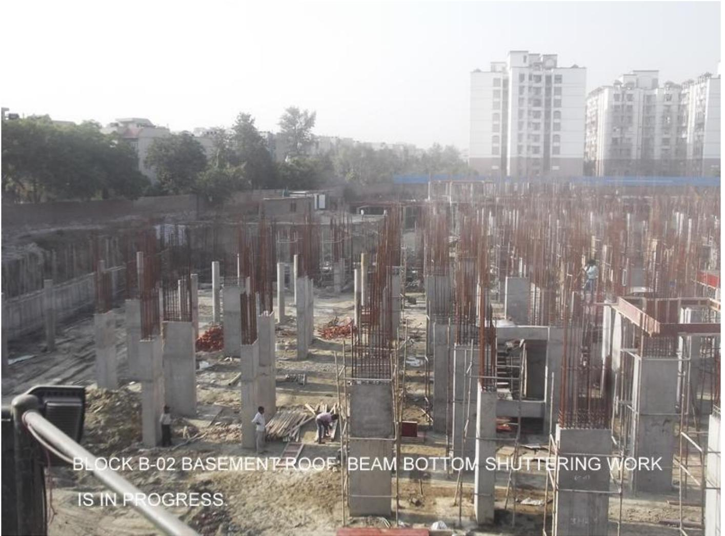
BLOCK B-02 BASEMENT ROOF BEAM BOTTOM SHUTTERING WORK
