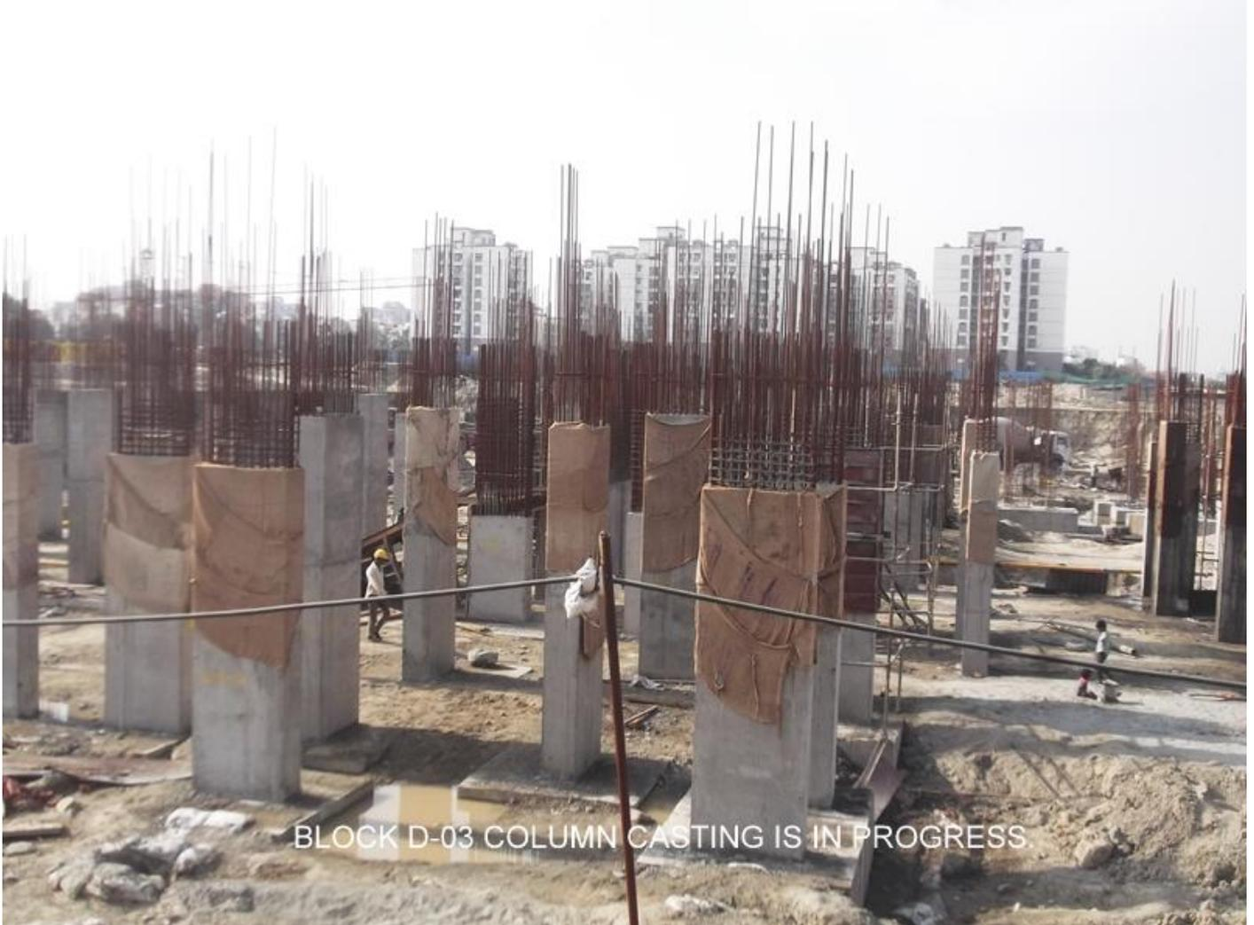
BLOCK D-03 COLUMN CASTING IS IN PROGRESS
