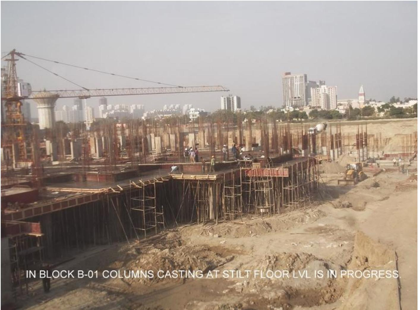
IN BLOCK B-01 COLUMNS CASTING AT STILT FLOOR LVL IS IN PROGRESS.
