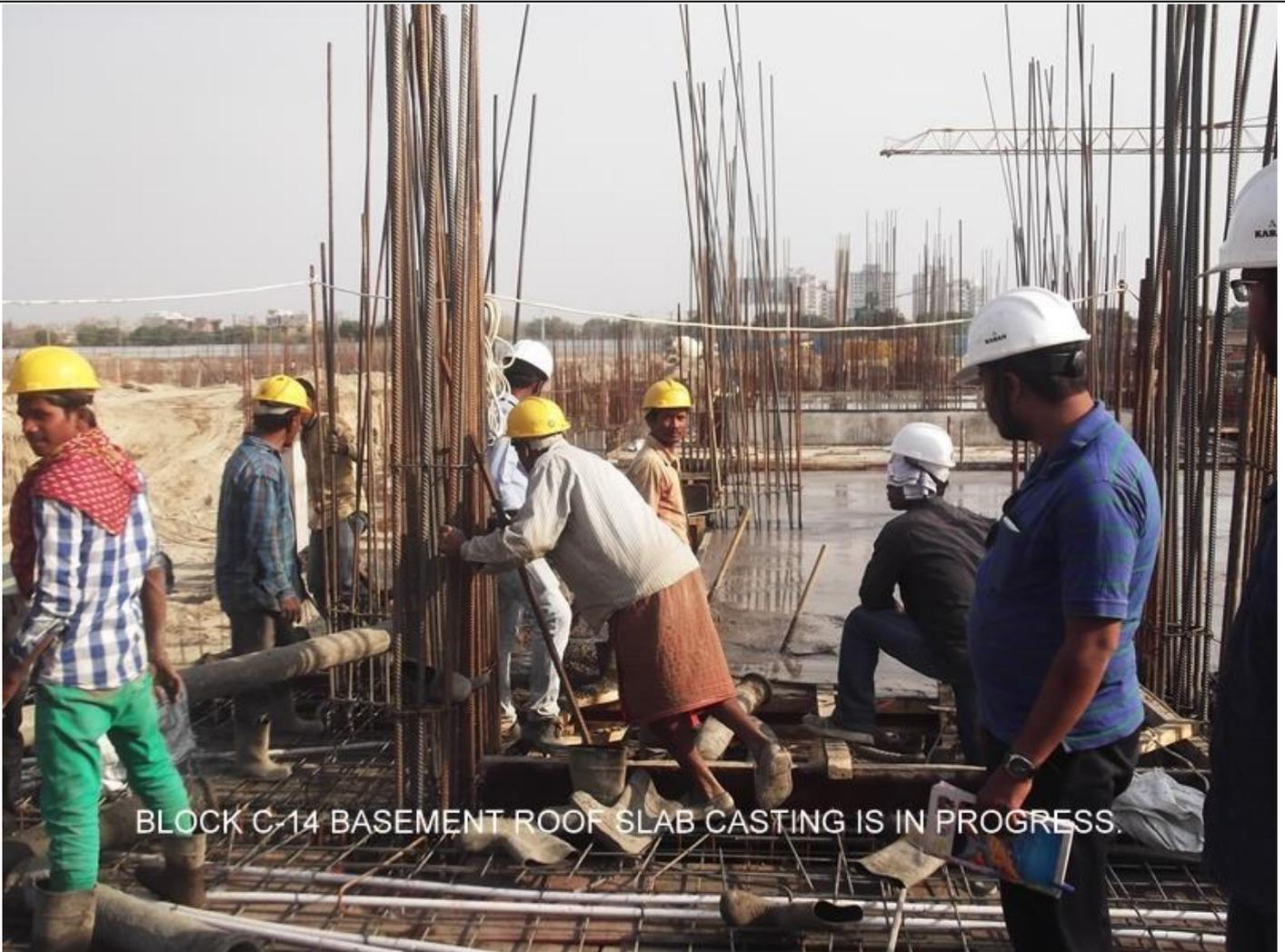
BLOCK C-14 BASEMENT ROOF SLAB CASTING IS IN PROGRESS.
